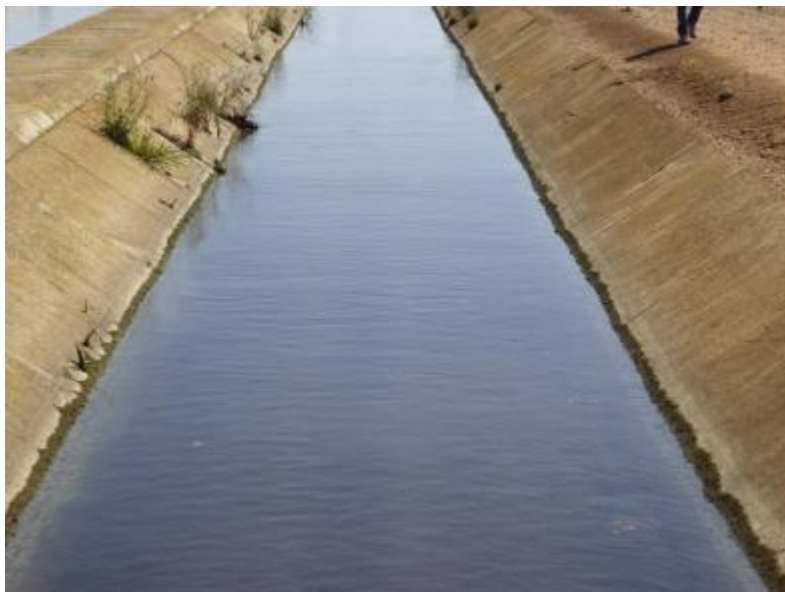
Figure 13. Canal transportant l'eau recyclée issue de Western Water (Source : Melbourne Water).
